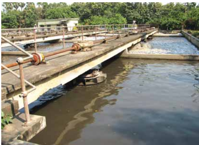
Fig-44. Sewage Treatment Plant (STP)
