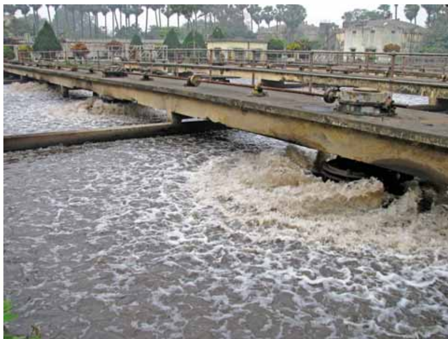
Fig-40. Aeration process in Sewage Treatment Plant
